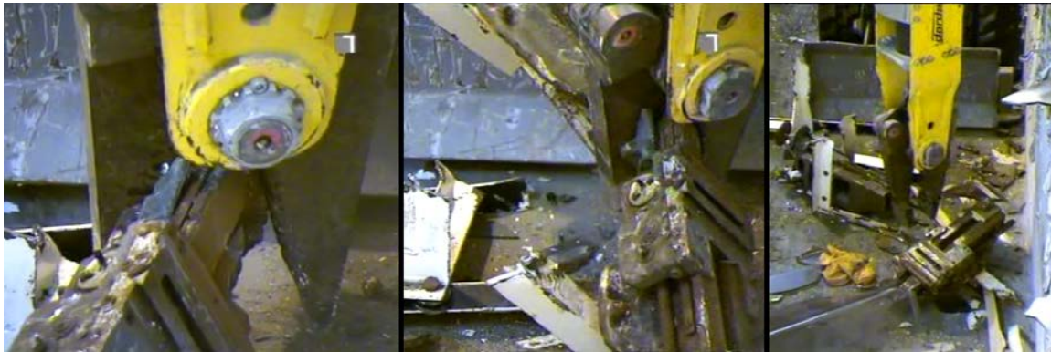
Figure 11 - Lathe being cropped by Darda HCS7 shear (CCTV stills)
