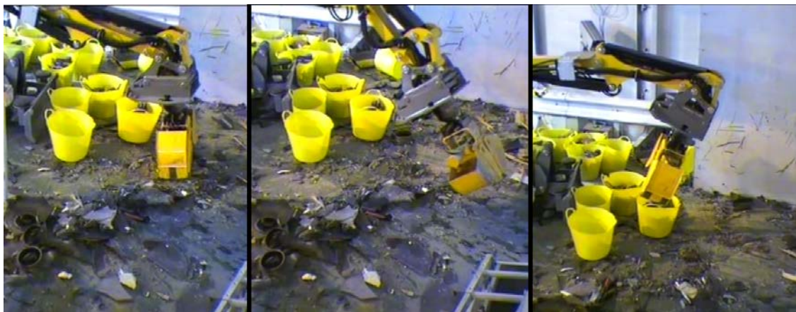
Figure 6 - Waste handling using C025H-25 clamshell bucket (CCTV stills)
