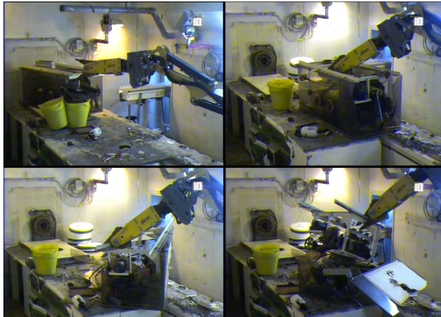
Figure 10 - Removal of internals from cutting cell glovebox (CCTV stills)
