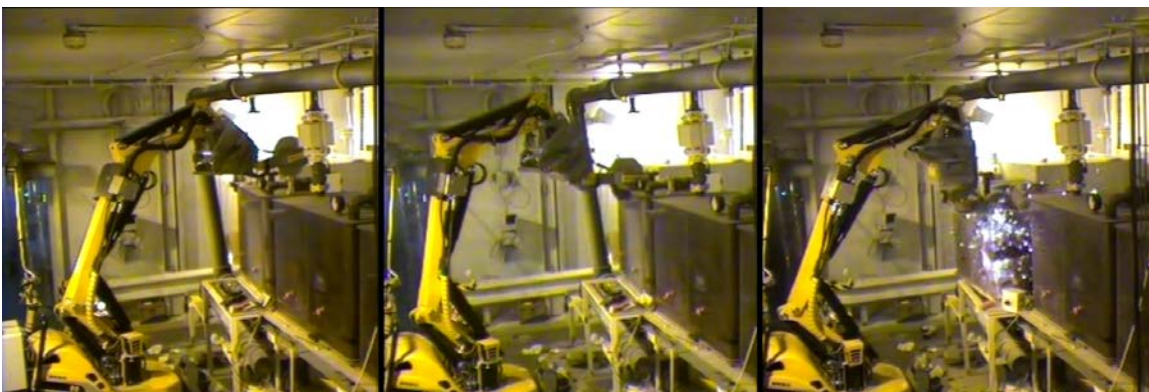
Figure 4 - Brokk® beginning size reduction of glovebox suite (CCTV stills)
