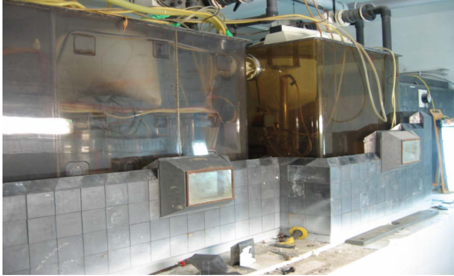
Figure 3 - Shielded section following partial lead removal
