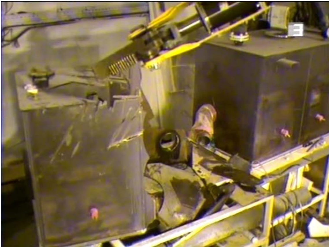
Figure 5 - Darda HCS7 shear being used to break up Darvic (CCTV still)
