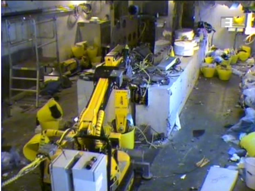
Figure 9 - General view of cell mid-decommissioning (CCTV still)
